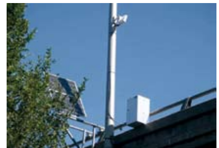
Wavetronics on bridge in Wichita.
