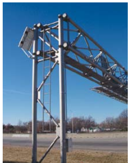
HD - Solar - truss.
